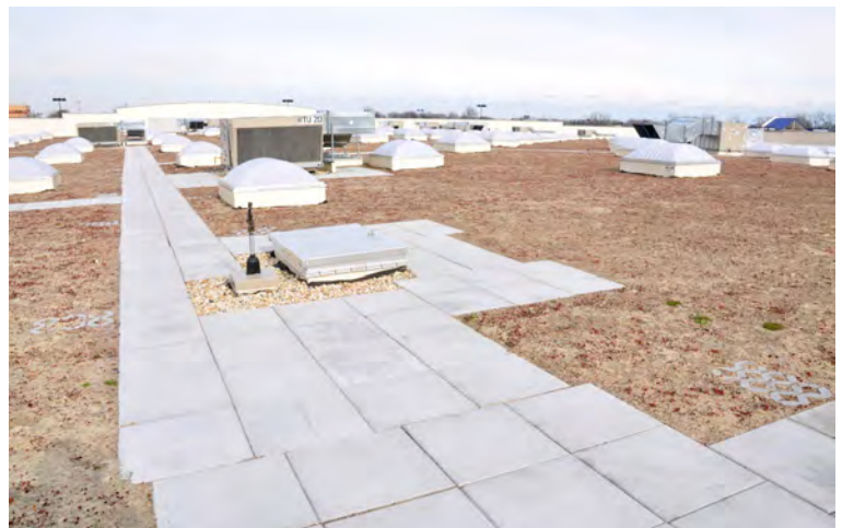
Using Wade's HydroMax siphonic roof drainage system, a Wal-Mart in Chatham, IL, reduced the number of large pipes needed from 14 to three, thus saving installation time and material costs. The system also allowed Wal-Mart to create a green roof.
